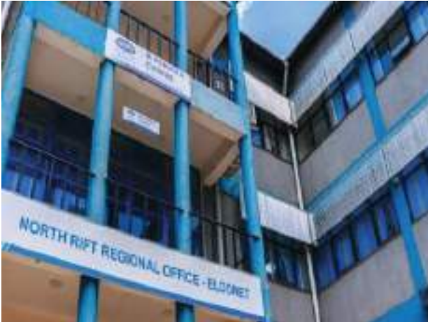
KEBS Eldoret Offices & Laboratories
