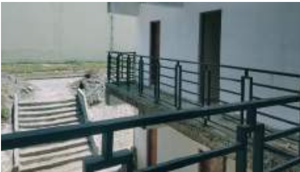
Infrastructure facilities at the Kenya Industrial Training Institute
