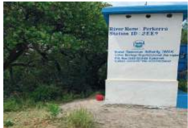
Telemetric Station constructed along Perkerra River
