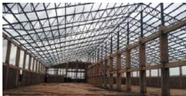
Status of factory building construction as of June 2022
