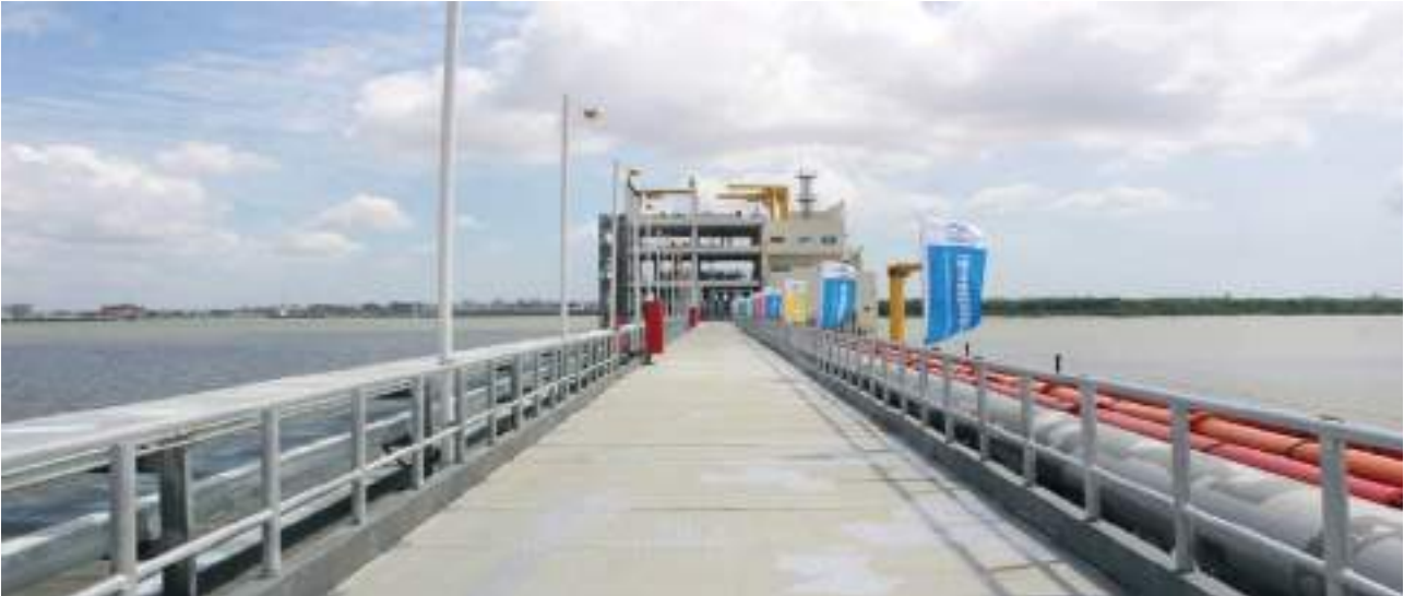
Relocated Kipevu Oil Terminal
