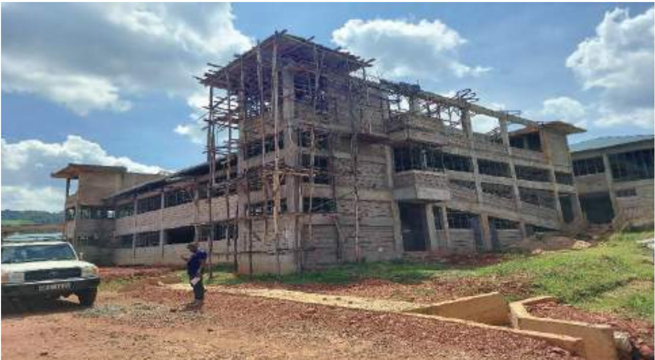
Ongoing Nyansiongo Market, Nyamira County
