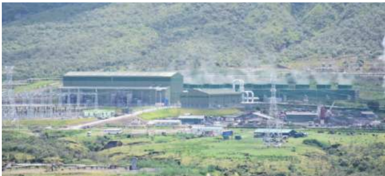
172.3MW Olkaria V Power Plant
