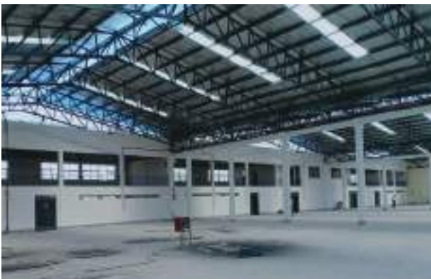
Industrial Shed in Cluster II
