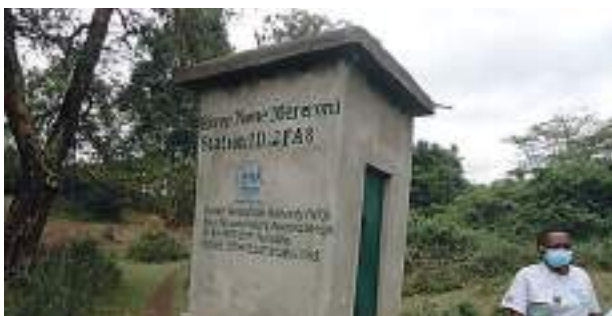
Well-Constructed Telemetric station housing along Mereroni Riverbank
