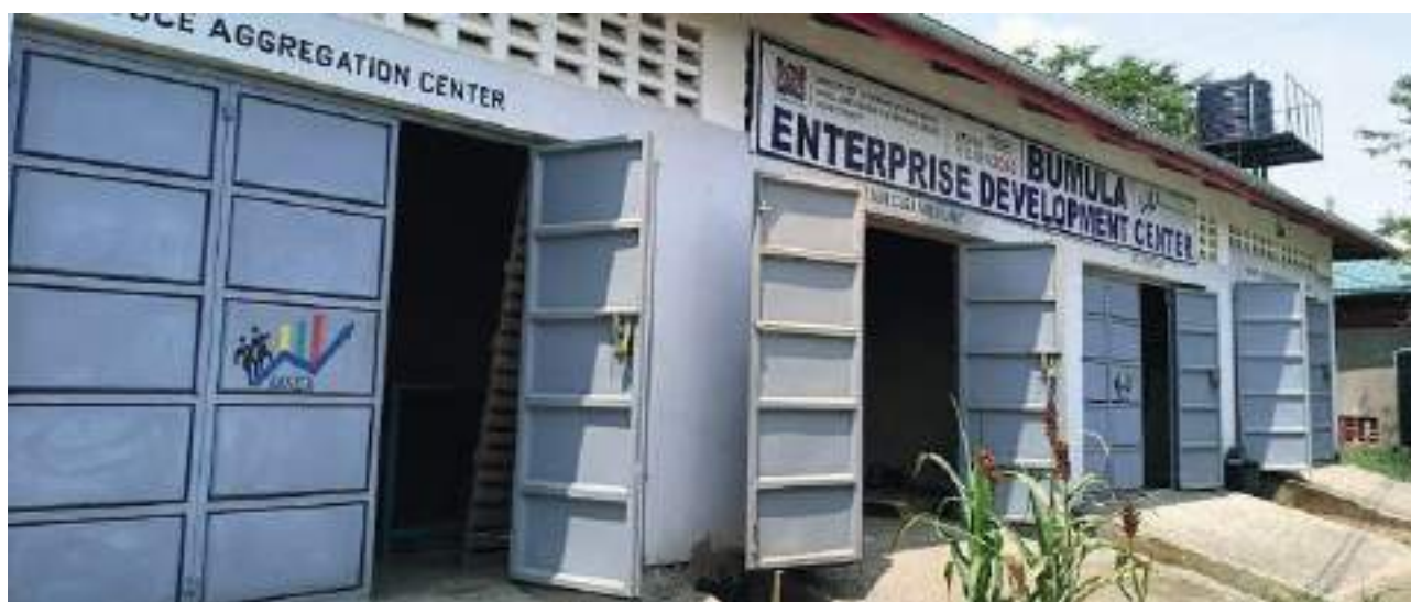
Refurbished and operationalised Constituency Industrial Development Centre in Bumala
