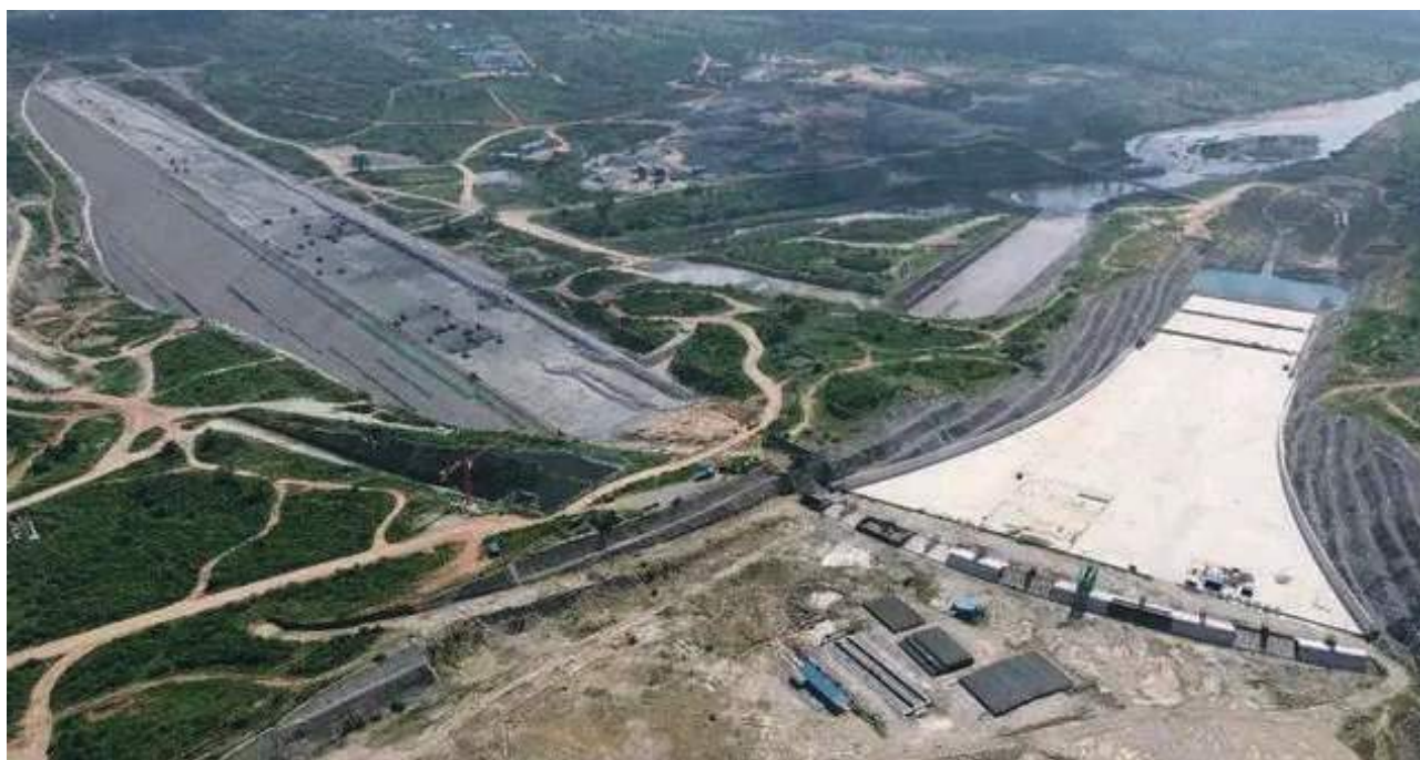
Thwake dam (70 percent) in Makueni/Kitui under construction
