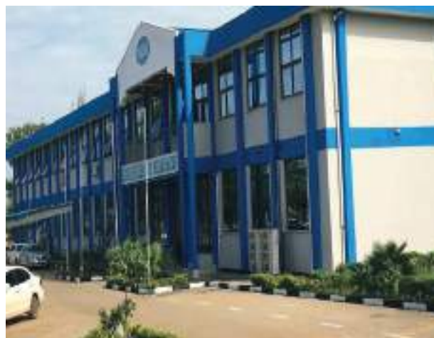
KEBS Kisumu Offices & Laboratories
