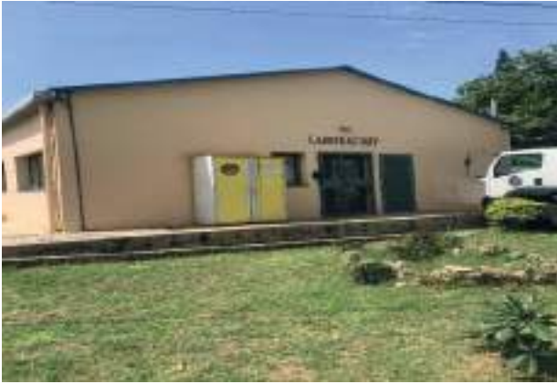
Completed Kisumu Fish Quality Laboratory
