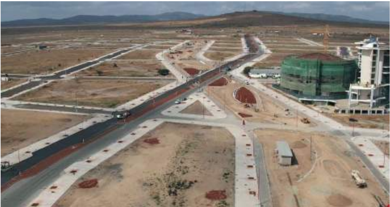
Konza Complex under construction.
