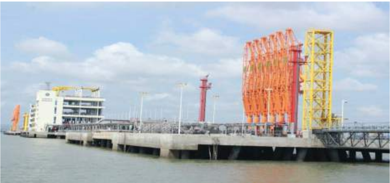
New Kipevu Oil Terminal
