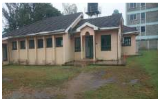
Completed Mombasa Fish Quality Laboratory
