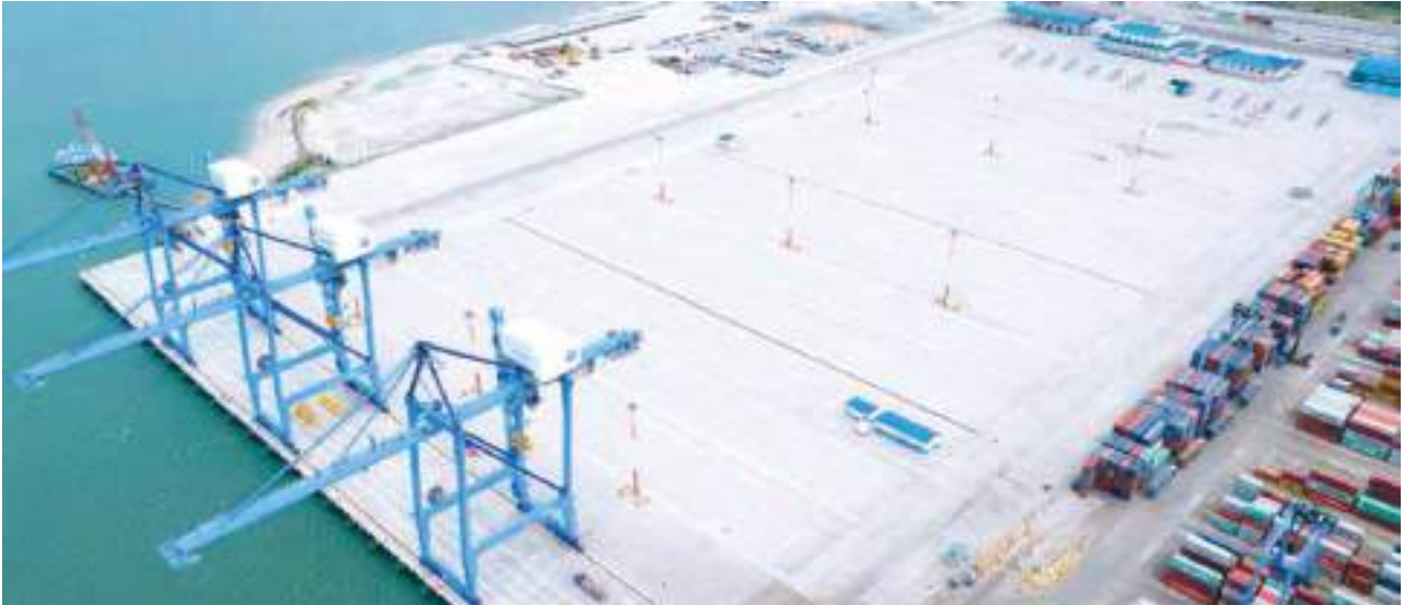
Aerial view of the completed Phase II of the Second Container Terminal
