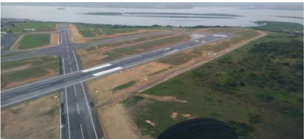
Pavement rehabilitated at MIA
