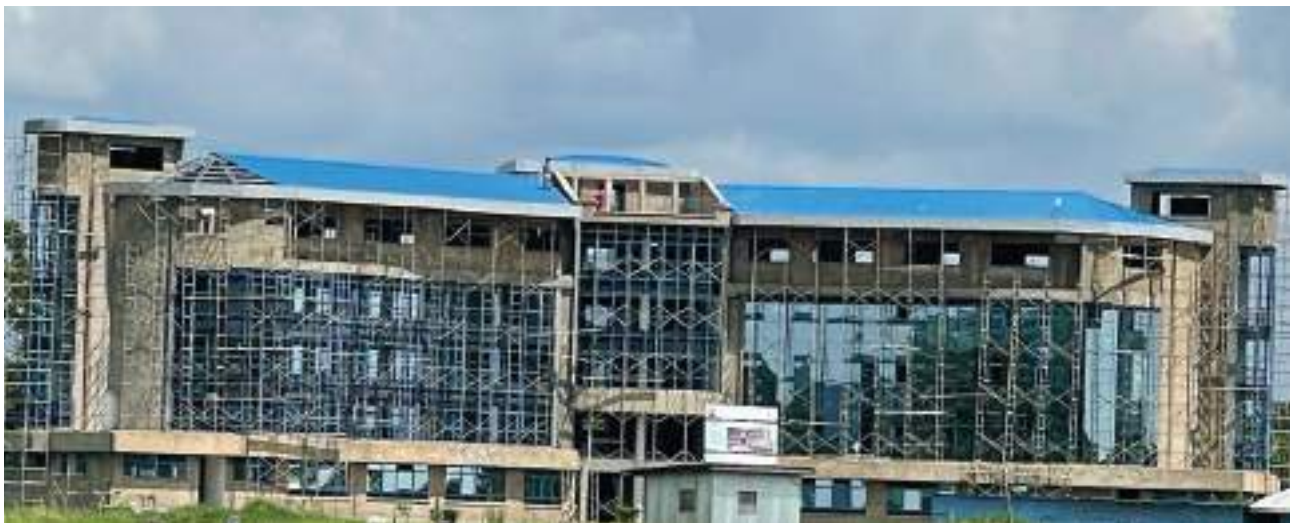
Front View of Sagana Aquaculture Facility under Construction
