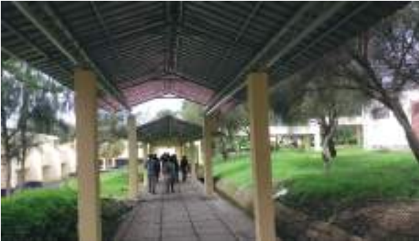
Infrastructure facilities (hostels, central stores, walkways, workshops) at KITI
