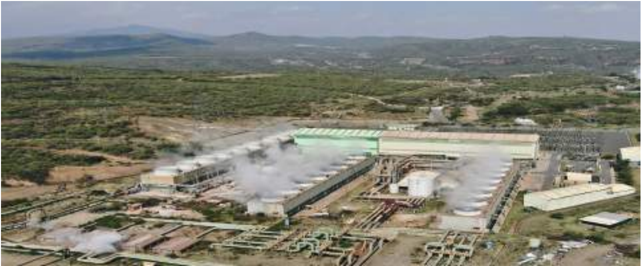
Olkaria I Unit 6 Power Plant
