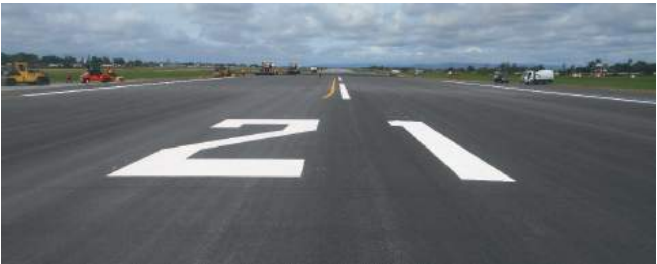
Runway rehabilitated at Moi International Airport
