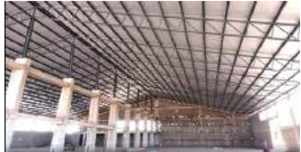
Oloitokitok Agro-Processing (Tomato) Plant Building
