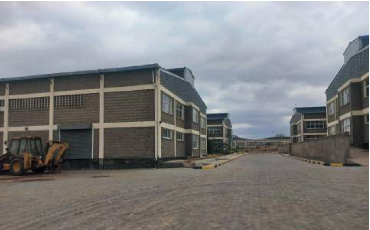
SME industrial sheds, Athi River EPZ
