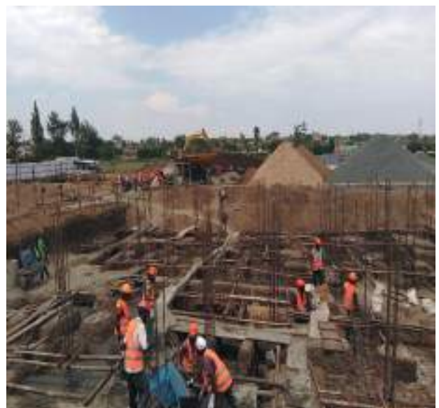
Kanyakwar Phase III, Kisumu County
