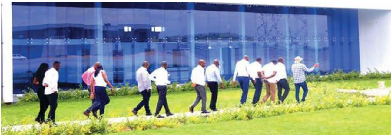
SEZA officials inspecting completion works at Africa Auto Auction (AAA) Jumbo SEZ Ltd building in Naivasha SEZ
