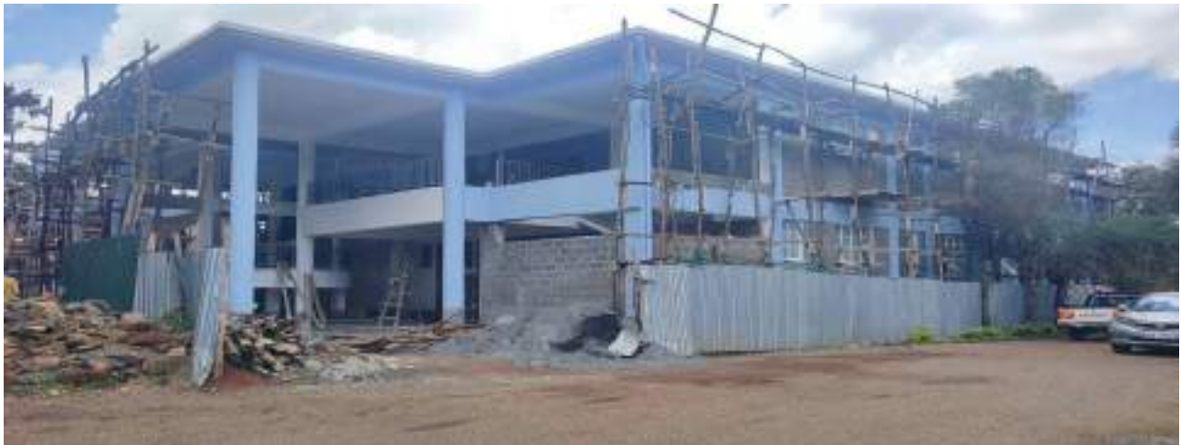
Construction of Cathlab
