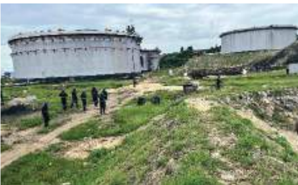
Tank auxiliary fittings
