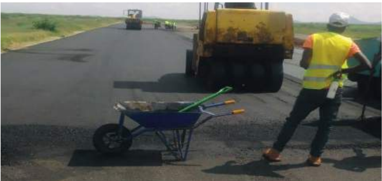
On-going rehabilitation and extension of runway at Isiolo International Airport
