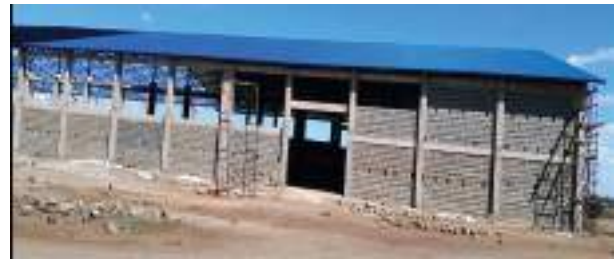
Oloitokitok Agro-Processing (Tomato) Plant Building
