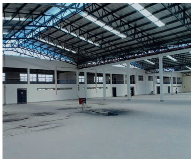
Industrial Shed in Cluster II
