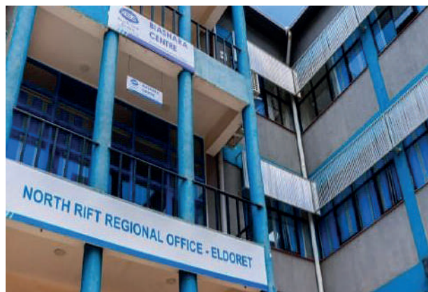
KEBS Eldoret Offices & Laboratories
