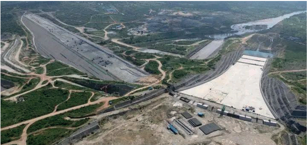
Thwake dam (70 percent) in Makueni/Kitui under construction
