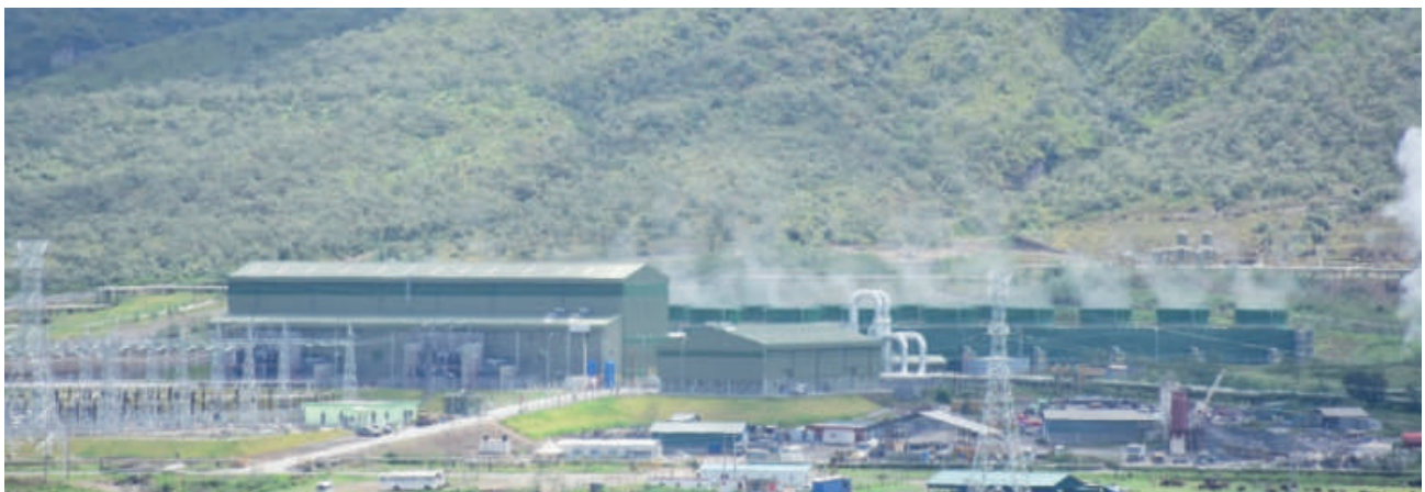
172.3MW Olkaria V Power Plant
