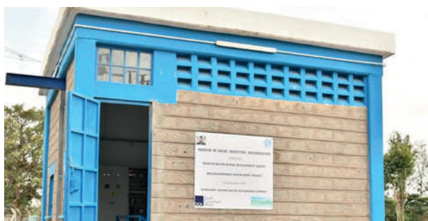
Completed Mavoko Drinking water supply Project in Machakos county.
