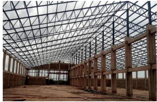
Status of factory building construction as of June 2022
