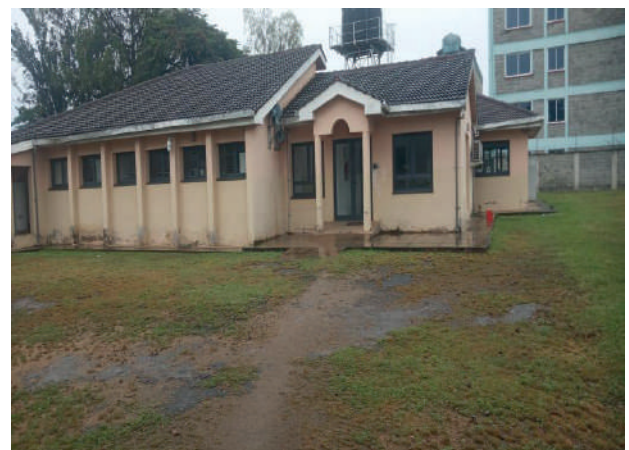
Completed Mombasa Fish Quality Laboratory
