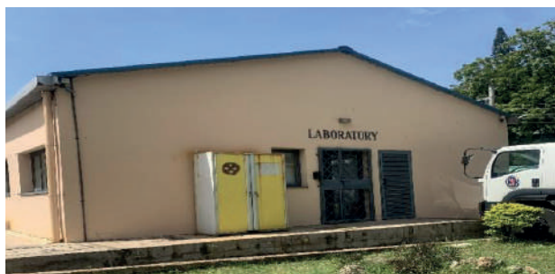
Completed Kisumu Fish Quality Laboratory
