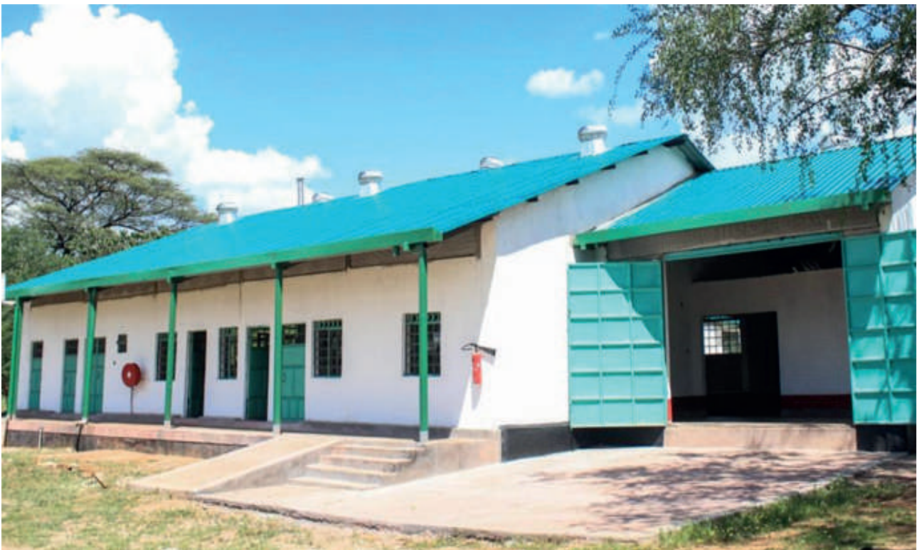
KVDA Mango Processing Factory in ToT, Elgeyo Marakwet
