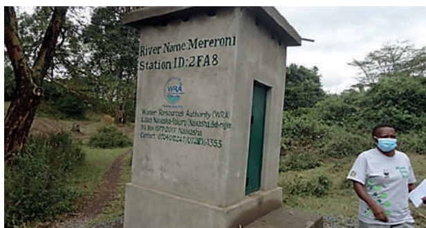
Well-Constructed Telemetric station housing along Mereroni Riverbank
