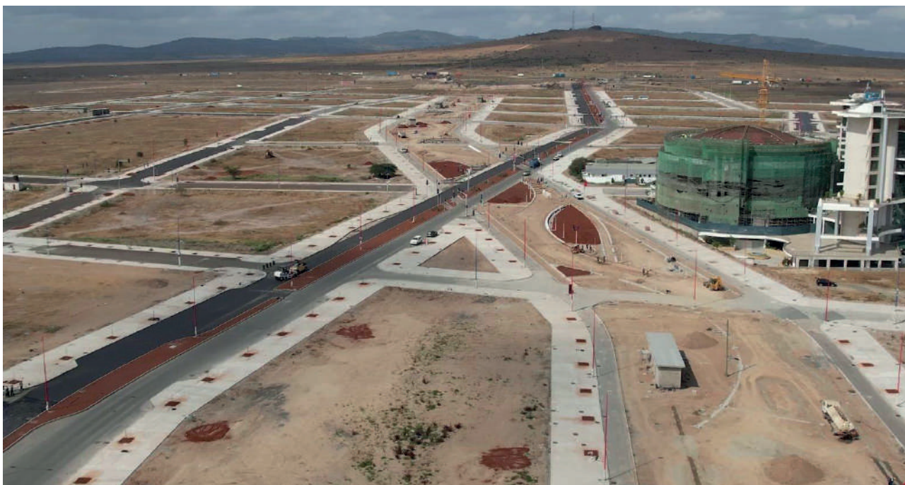
Konza Complex under construction.
