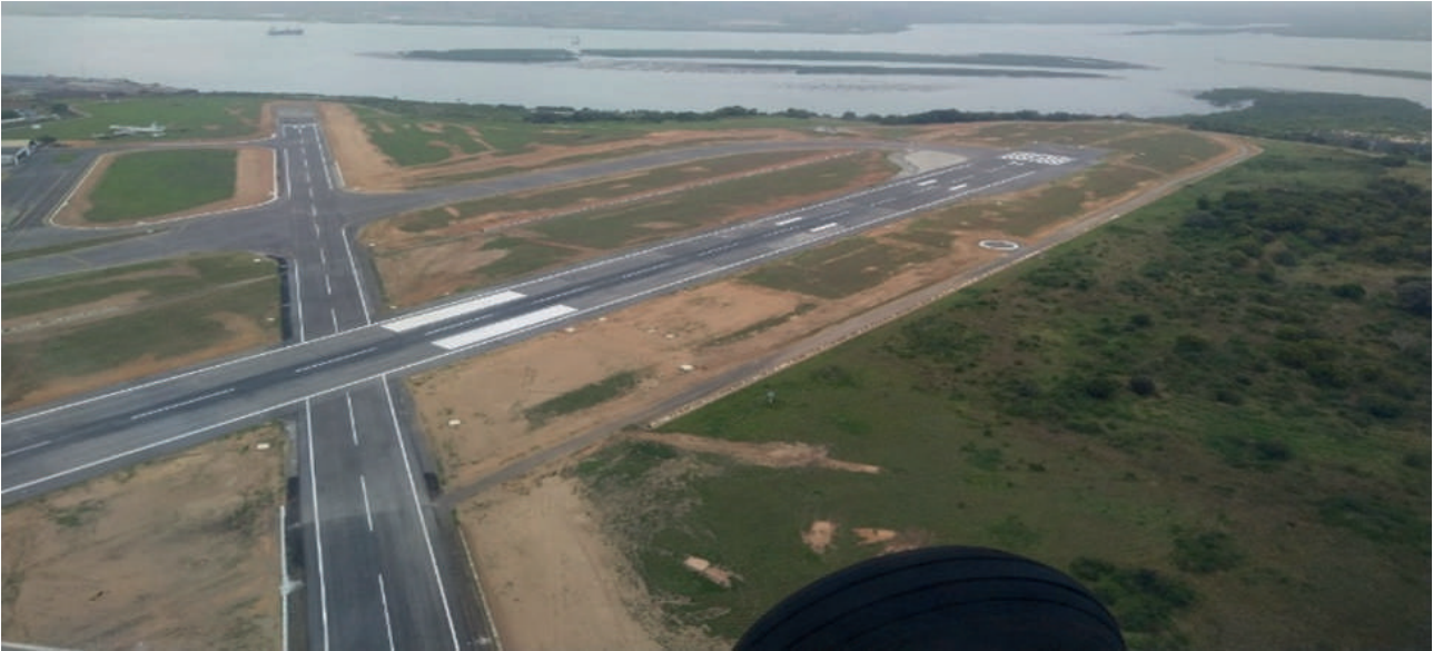
Pavement rehabilitated at MIA
