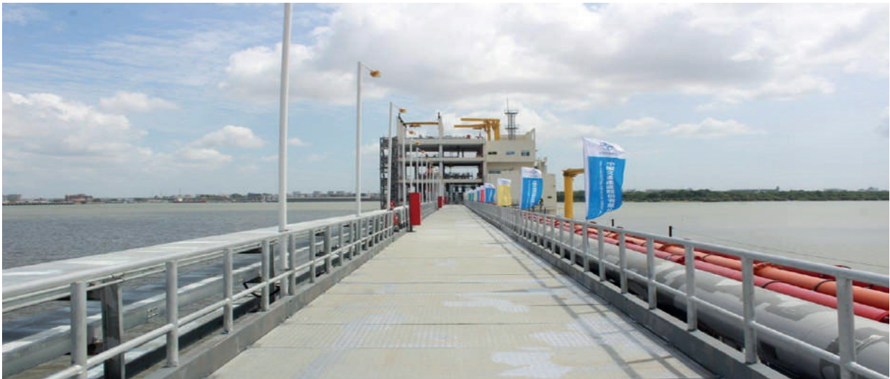
Relocated Kipevu Oil Terminal
