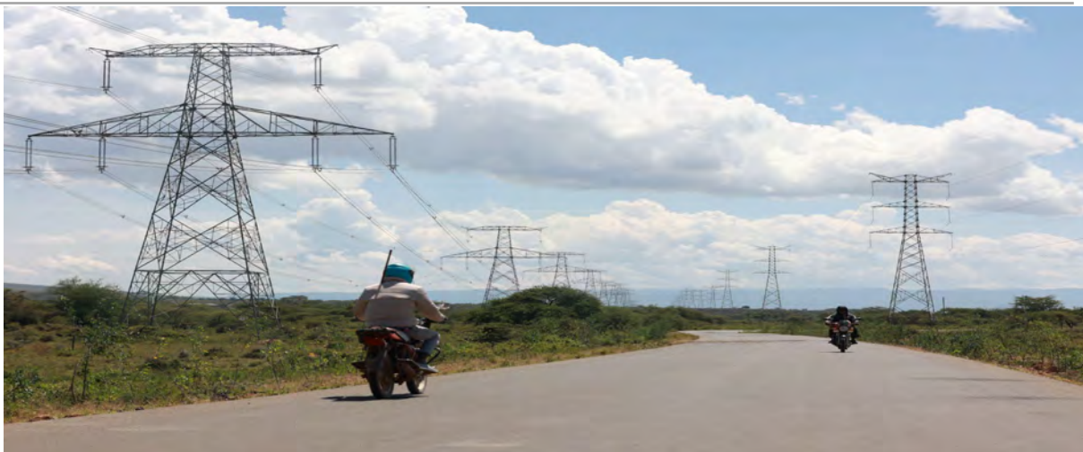
Transmission Lines from Suswa Sub-Station to Kimuka Sub-Station crossing at Kimuka Suswa Road
